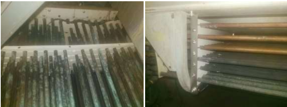
Figure 2: Field installation of retrofit kit
